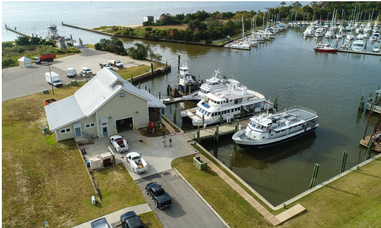
Figure 5: The Marine Maintenance Facility at Deep Point
