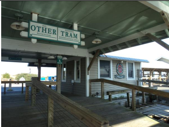
Covered Passenger Deck
