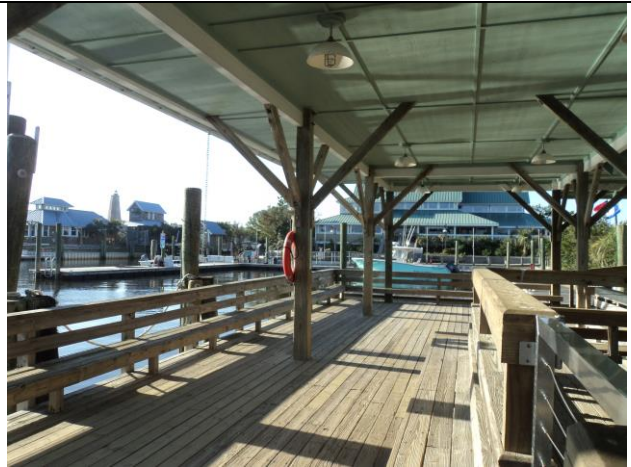
Covered Passenger Deck
