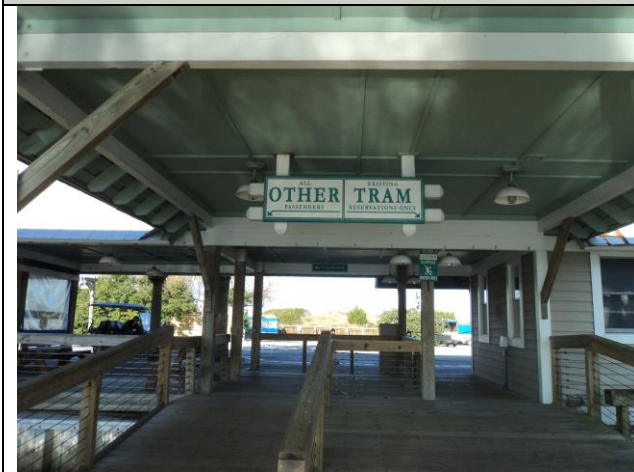
Covered Passenger Deck
