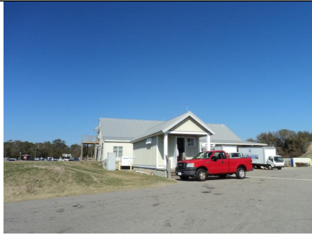
Computer Server Building
