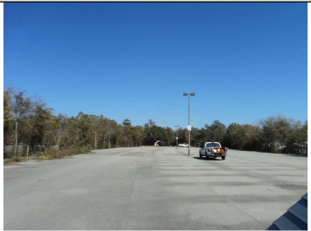
Typical Parking Area
