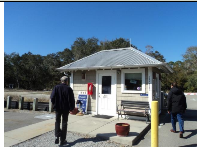
Typical Parking Attendant Station
