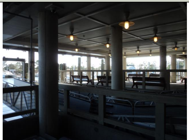
Passenger Waiting Area
