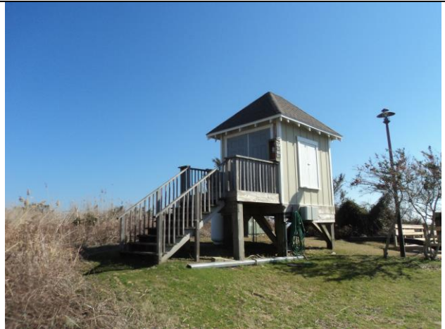
Barge Lift Mechanical Building
