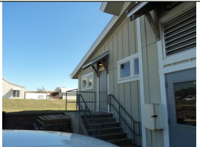
Ferry Repair Building
