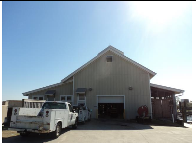
Ferry Repair Building
