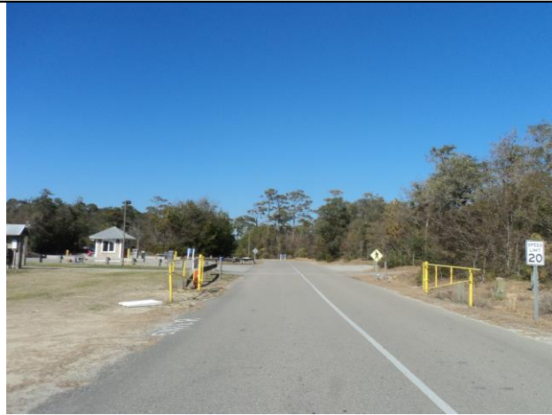
Typical Access Road
