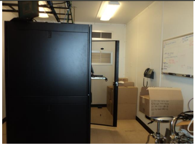
Computer Server Building
