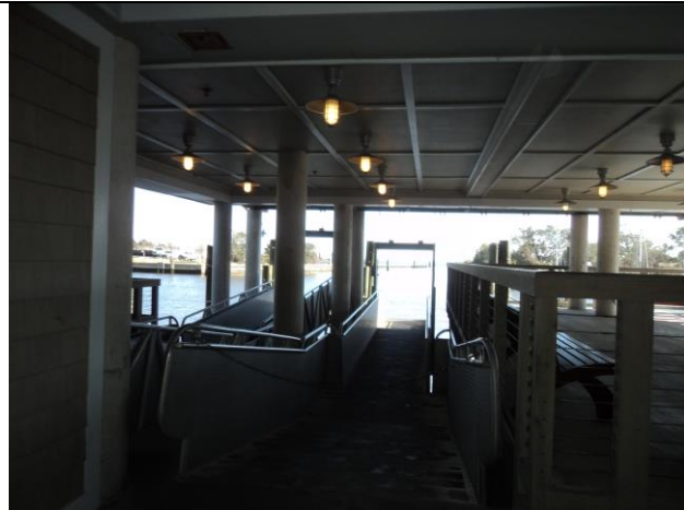
Passenger Boarding area
