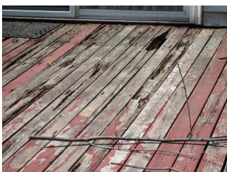
Split or decaying wood: Check several areas, pay attention to damp areas
