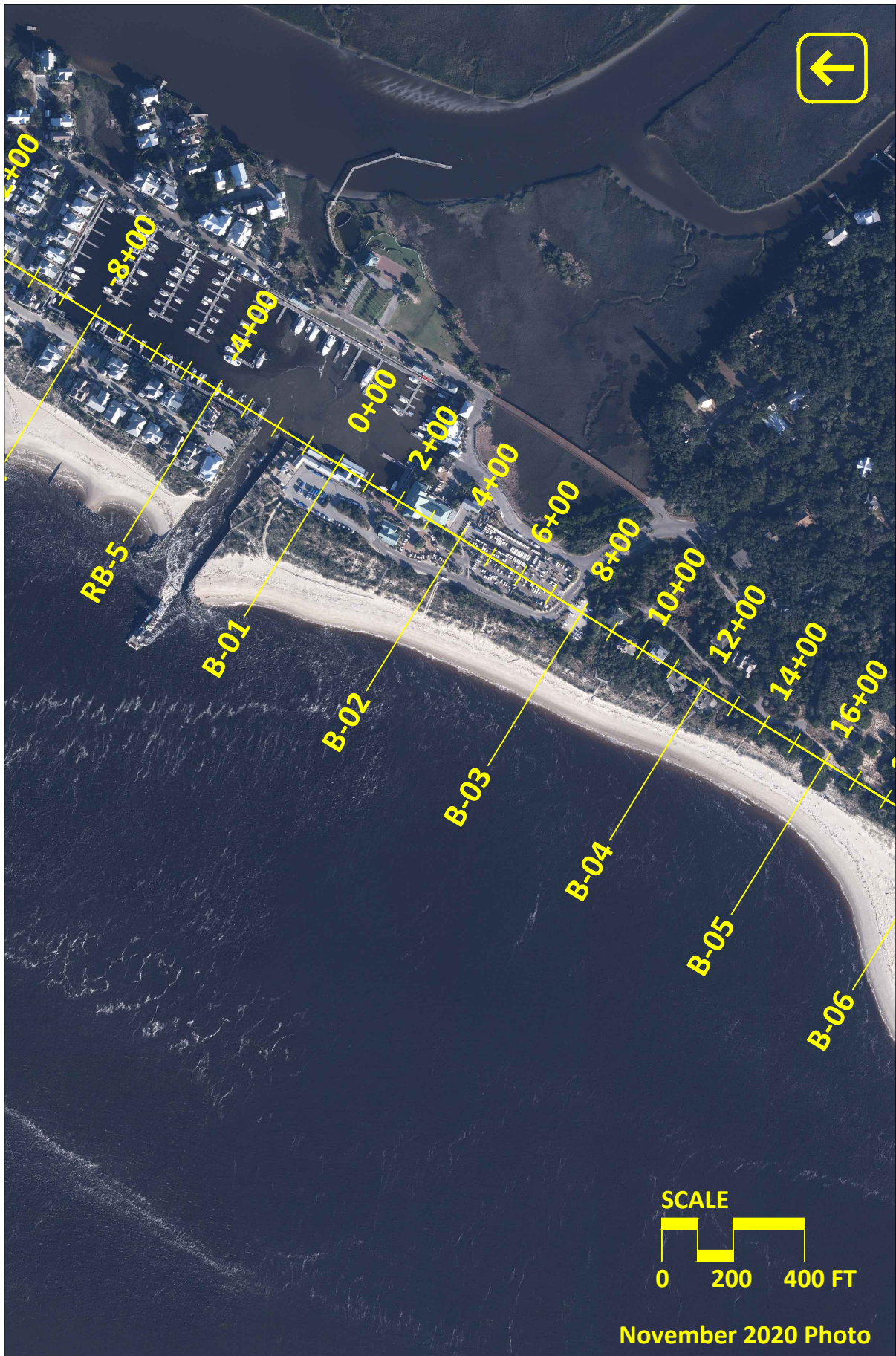
Figure C-3: Bald Head Island November 2020 aerial photography.
