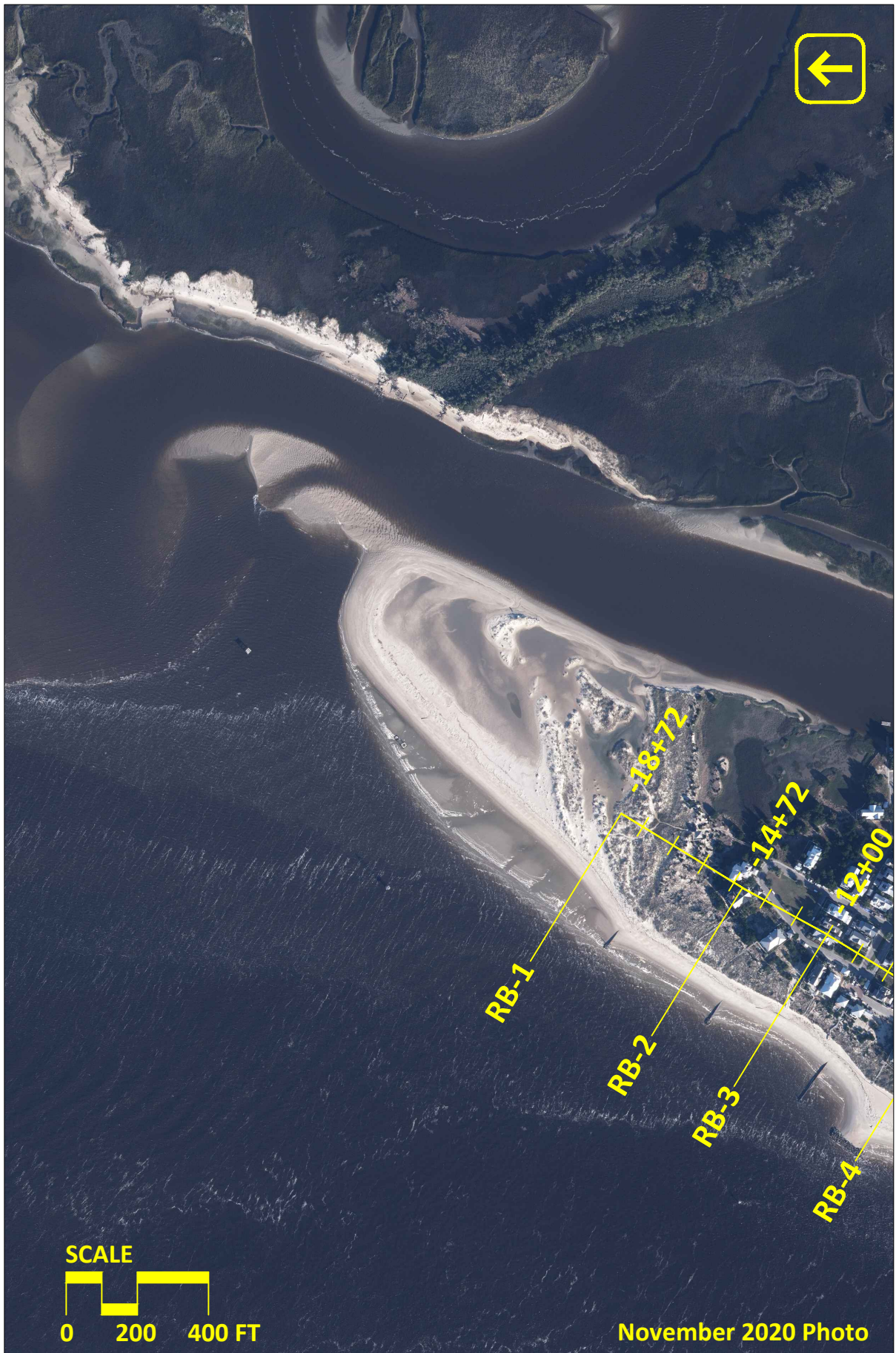
Figure C-2: Bald Head Island November 2020 aerial photography.
