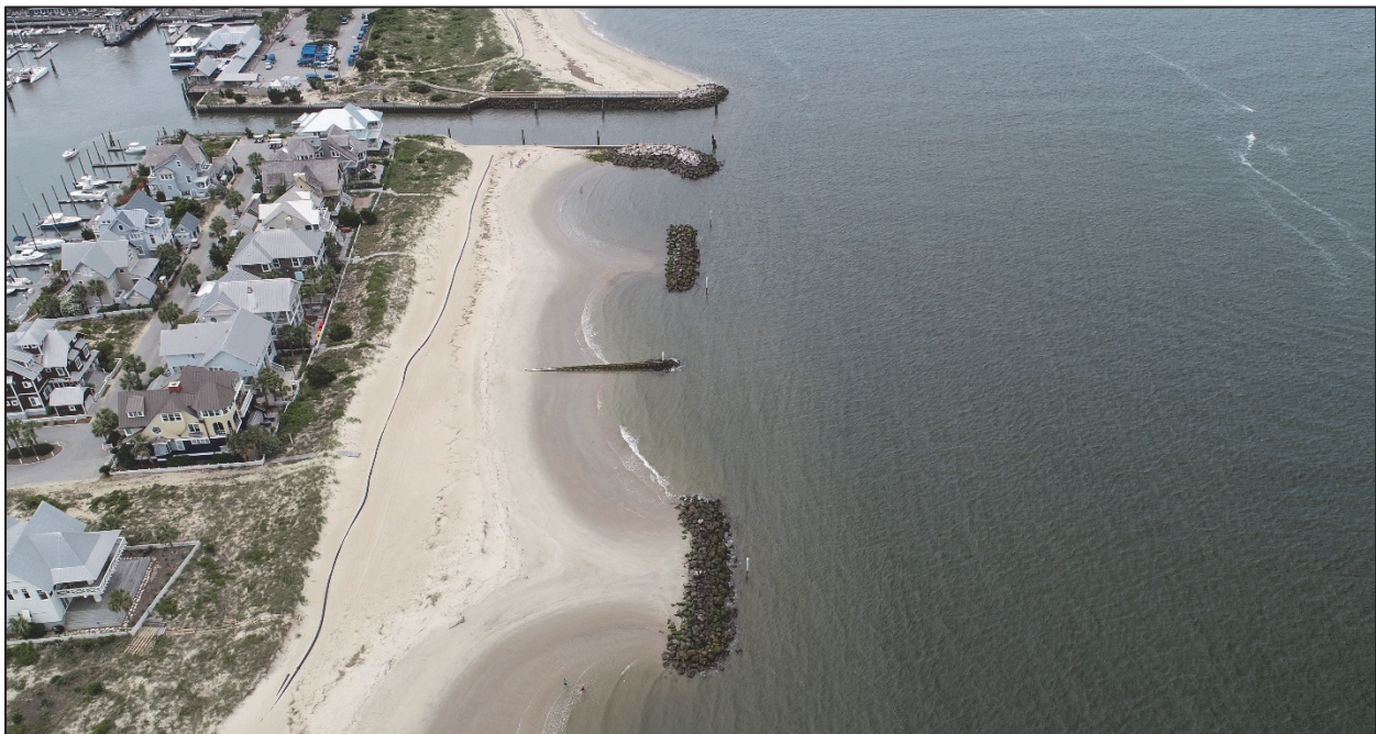
Figure 3.11: Southward looking view of the Row-Boat-Row shoreline detached breakwaters (June 2021 photo).
