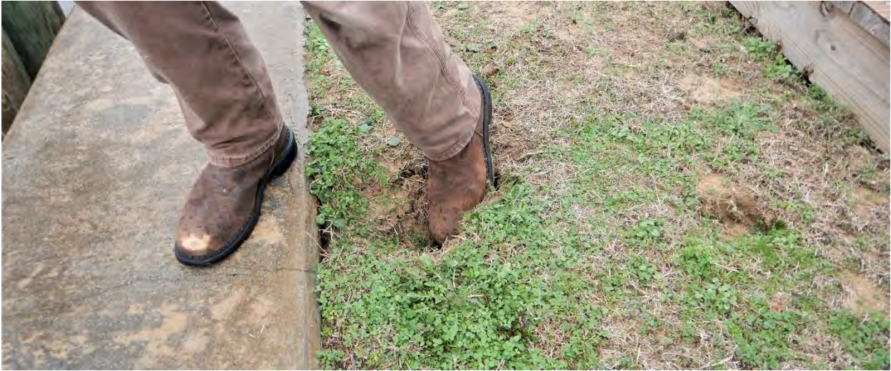
FIGURE 2-15: TYPICAL SINKHOLES BEHIND WALL
