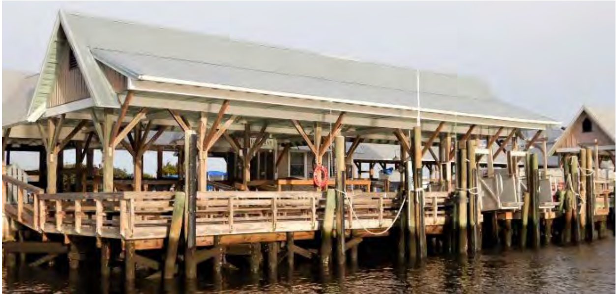
FIGURE 2-25: BHI PASSENGER LANDING UNDERDECK VIEW (LOOKING EAST)
