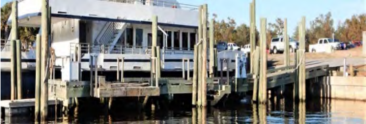
FIGURE 2-6: DPM MAINTENANCE FIXED PIER TIMBER PILE BENTS
