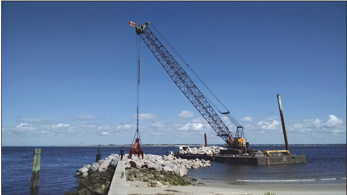
Figure 1.14: New rock placement at the North Jetty, Bald Head Island marina (May 29, 2015).
