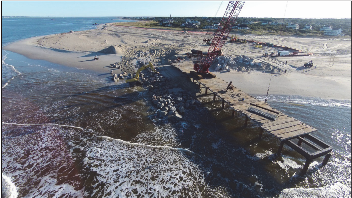
Figure 1.7: Rock and mattress placement along seaward end of terminal groin utilizing a temporary trestle structure (October 22, 2015).
