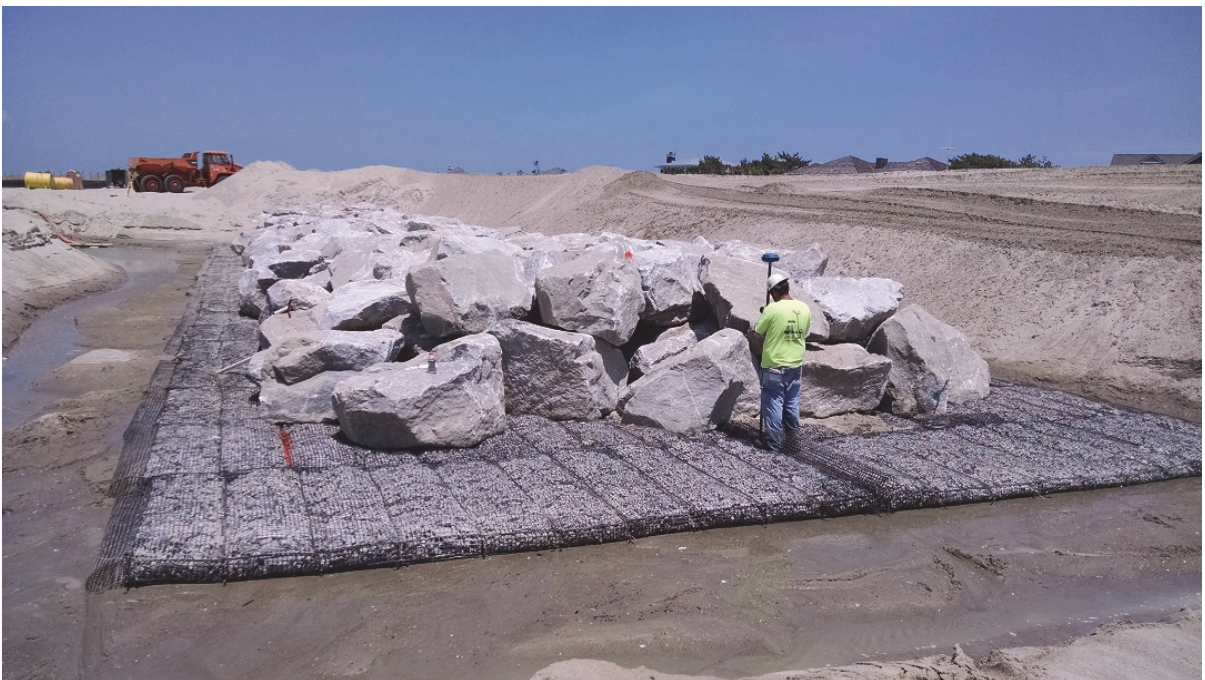
Figure 1.6: Rock and mattress placement verification (July 21, 2015).
