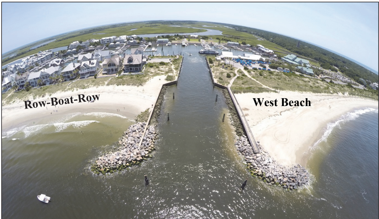
Figure 1.15: Completed jetty extensions at the Bald Head Island marina (July 12, 2015).
