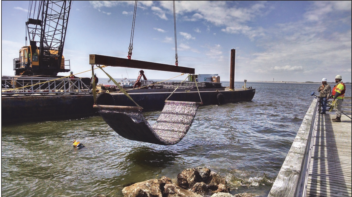
Figure 1.12: Laying of the first mattress for the south jetty extension at the Bald Head Island marina (March 25, 2015).
