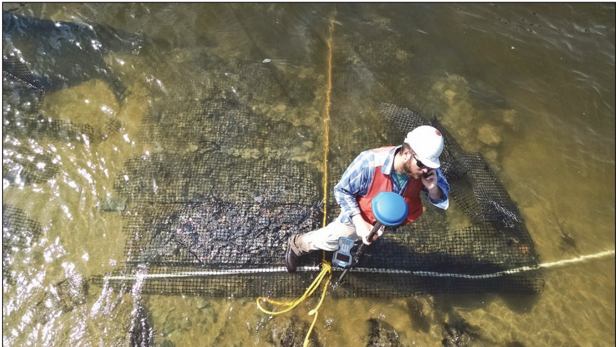
Figure 1.13: Location verification of placed mattress, Bald Head Island marina (April 6, 2015).
