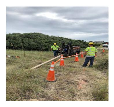
We appreciate the community's patience and support as we continue this work in 2022. Above is an example of crews working to install new underground power lines with specialty equipment to minimize open digging.
