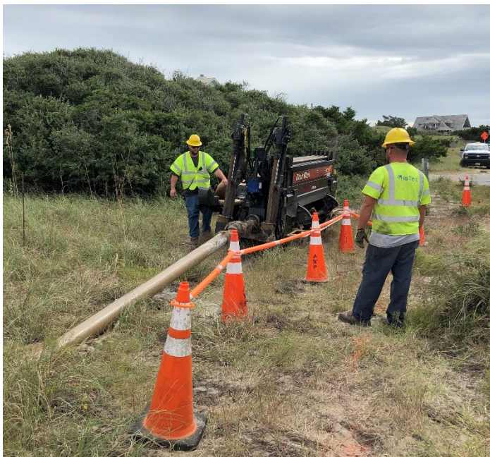
Crews working to install new underground power lines with specialty equipment to minimize open digging.
