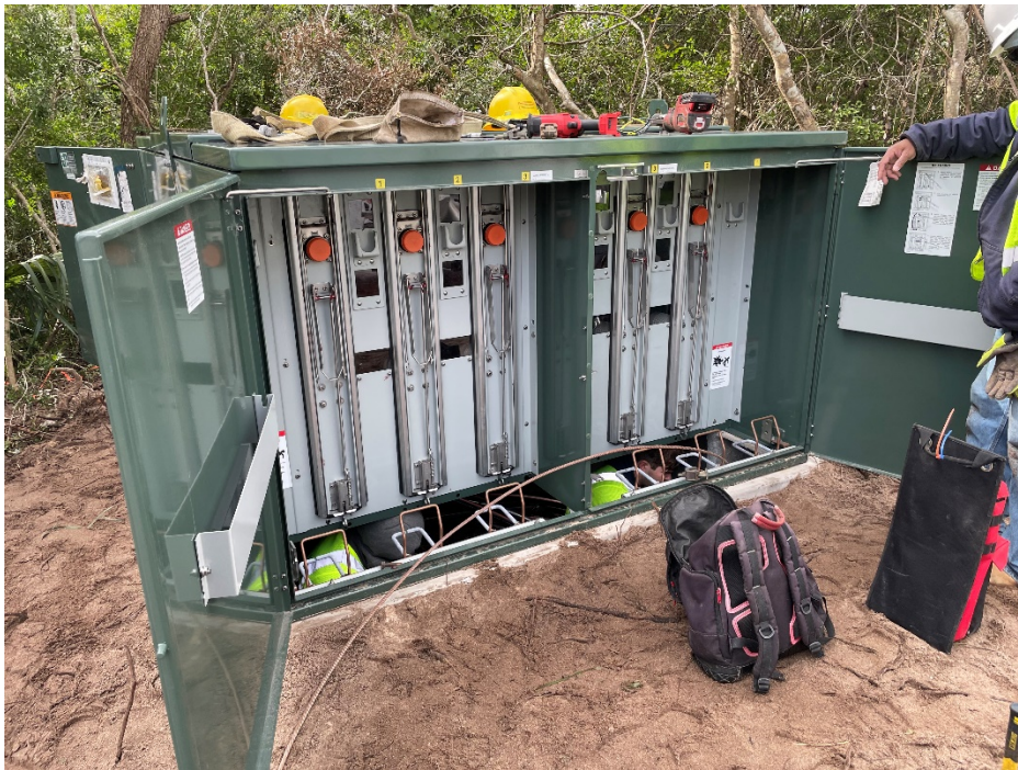
New underground switch installed along Federal Road last week.
