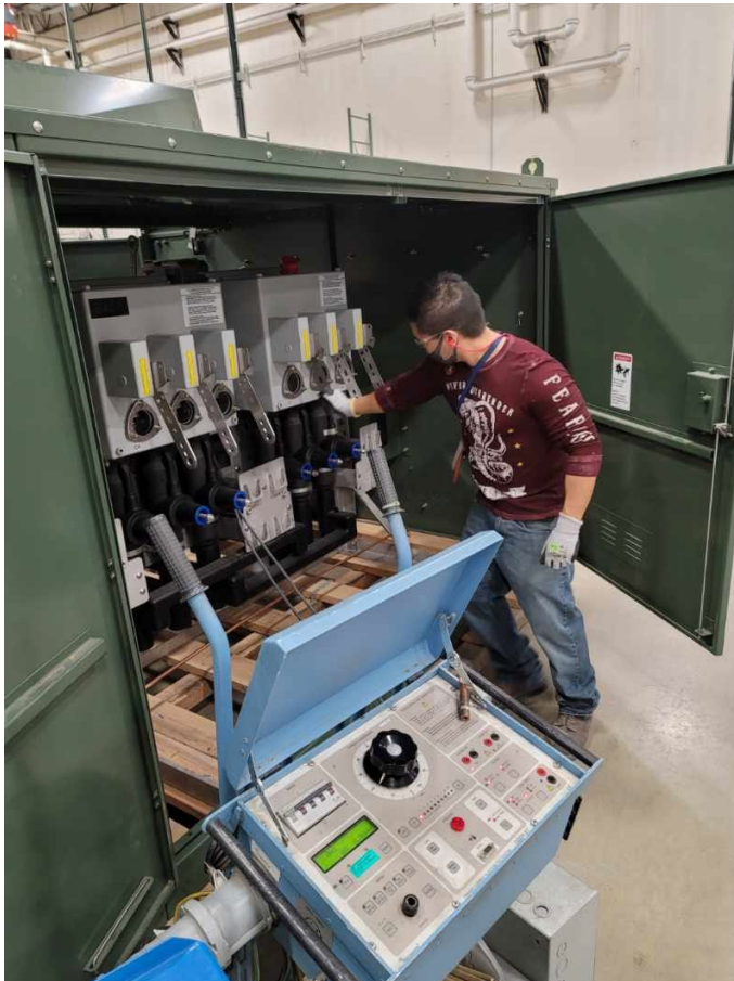
New custom underground switch being tested at the manufacturing facility.
