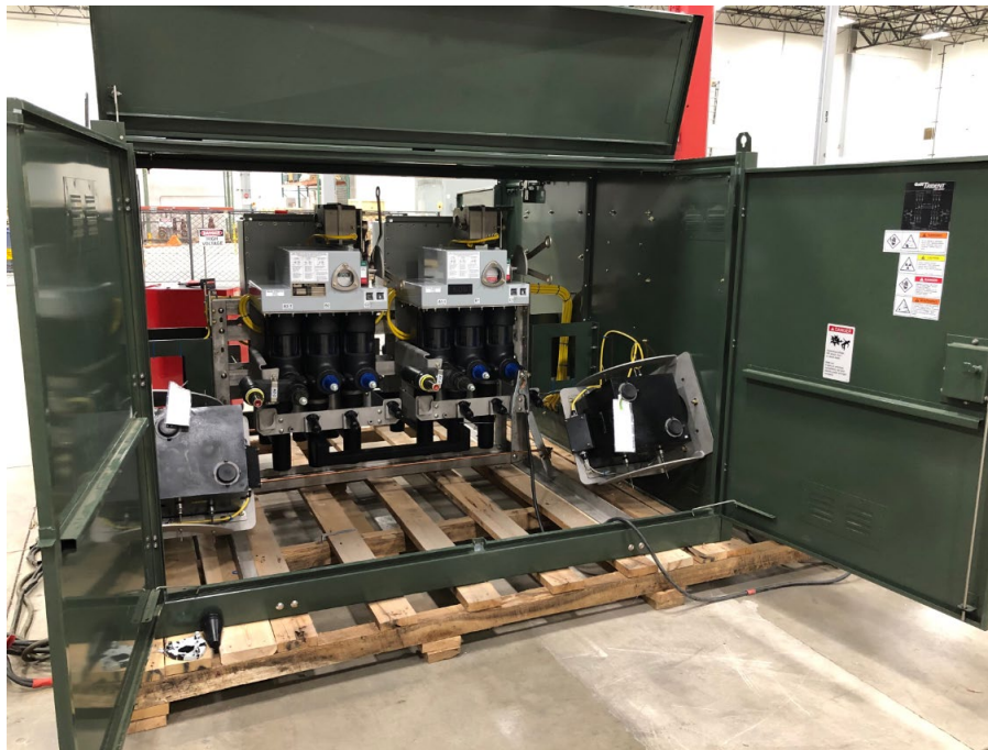
Custom manufactured switchgear being tested at the manufacturing facility in Ohio before being shipped to North Carolina.
