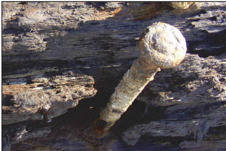
Figure 14. Example of shelf clamp bolt with washer.
