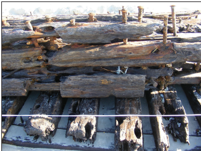
Figure 8. Shelf timbers and associated deck beam rebates.
