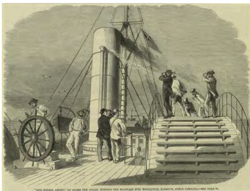
Figure 14. July 1864 image of the deck of the blockade runner Lilian running into Wilmington (courtesy of the NYPL).
