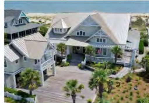
Single family homes are the predominant land use in the village. For many of the homeowners, these are vacation homes, not their primary residences.
