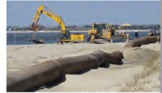
Beach renourishment and channel dredging are two key island management activities.
