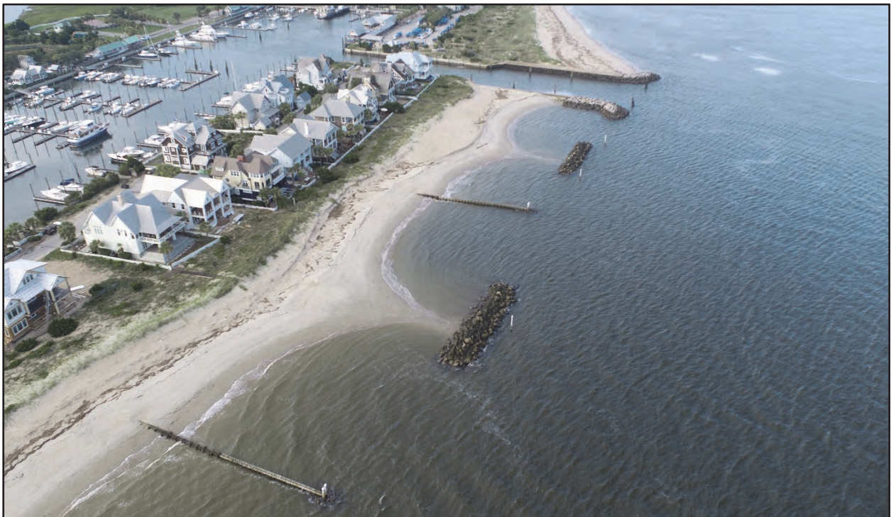
Figure 3.13: Southward looking view of the Row-Boat-Row shoreline detached breakwaters (July 2023 photo).
