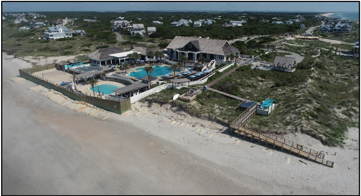
Figure 4: Sandbag revetment placed in front of the Club in June 2022. Photo from July 2023.
