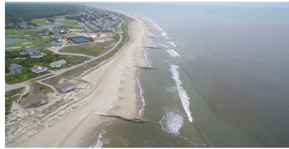
The Bald Head Island groin field consists of 13 sand-filled geotextile tubes extending seaward from the beach. Photo: Village of Bald Head Island
