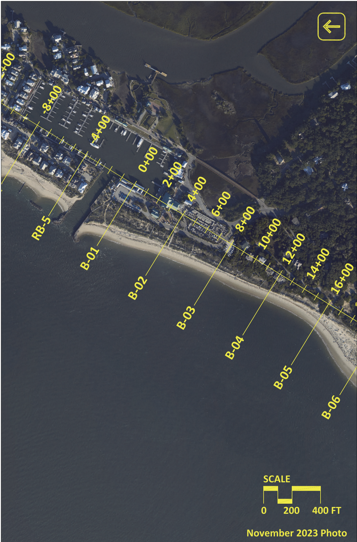
Figure C-3: Bald Head Island November 2023 aerial photography.
