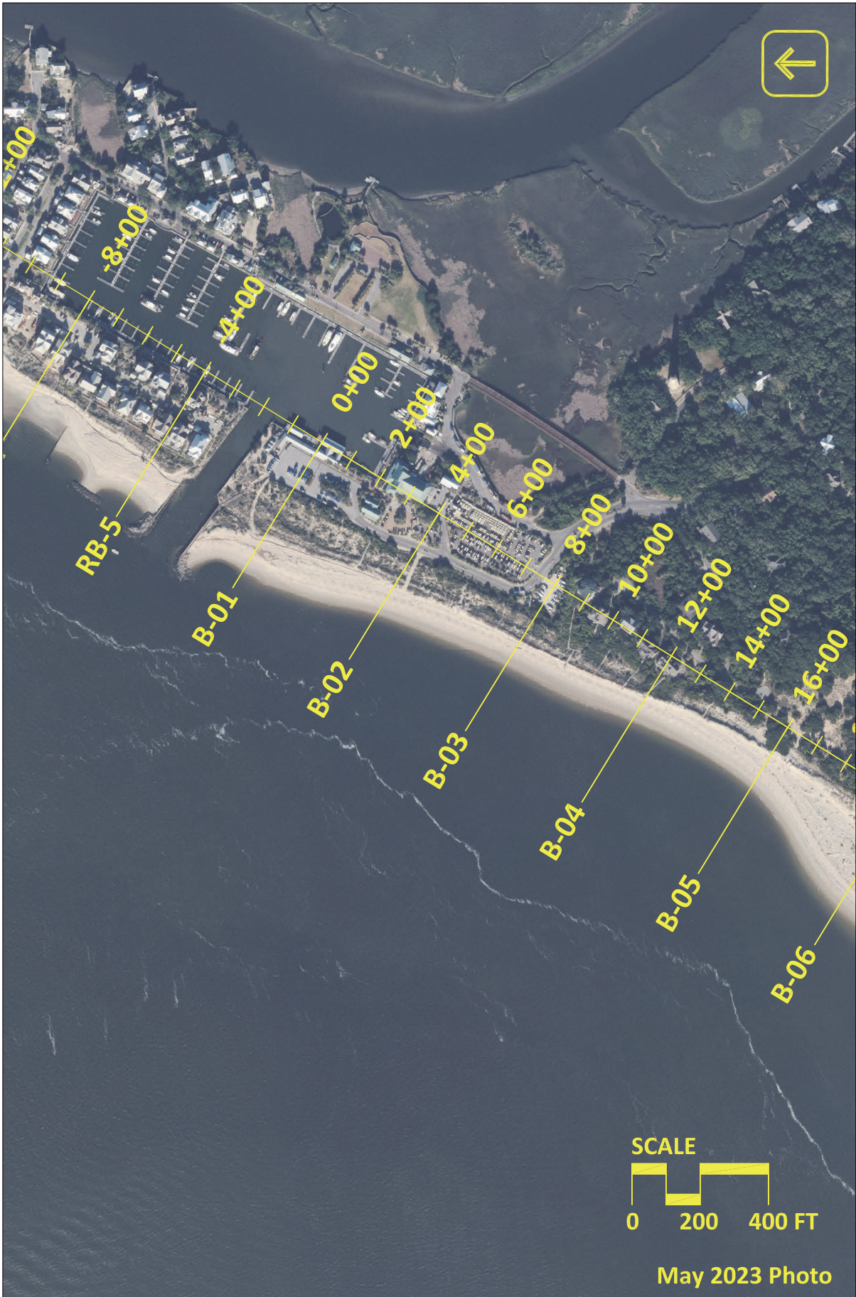
Figure D-3: Bald Head Island May 2023 aerial photography.
