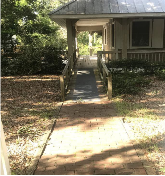
Accessible Ramp to Village Hall
