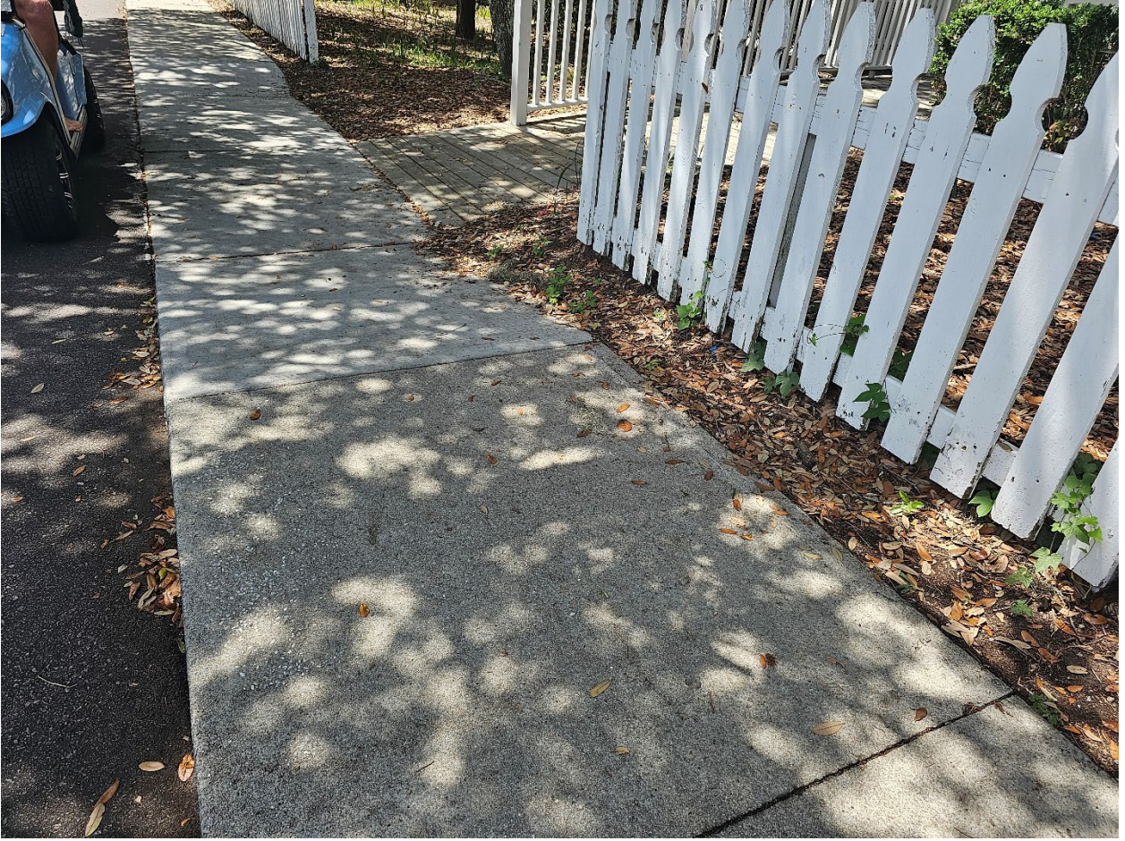
Area Where Curb cut was installed.
