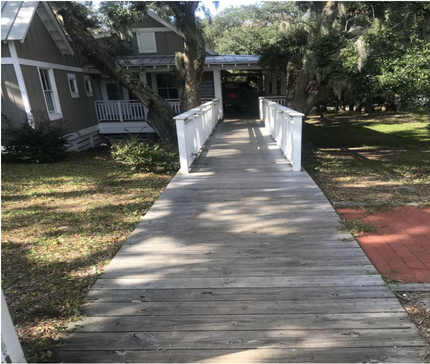
Ramp to side entrance
