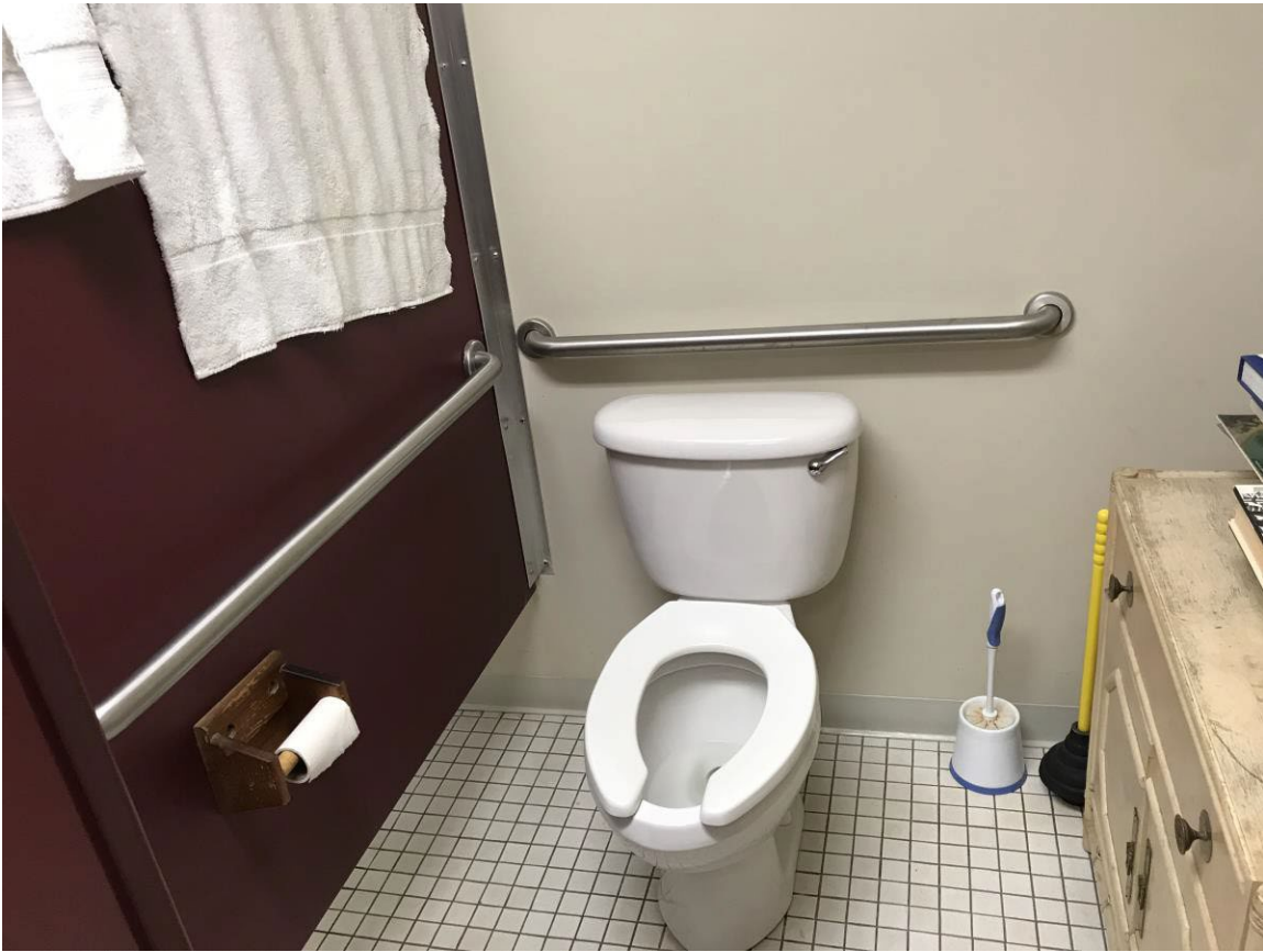
Toilet area with grab bars
