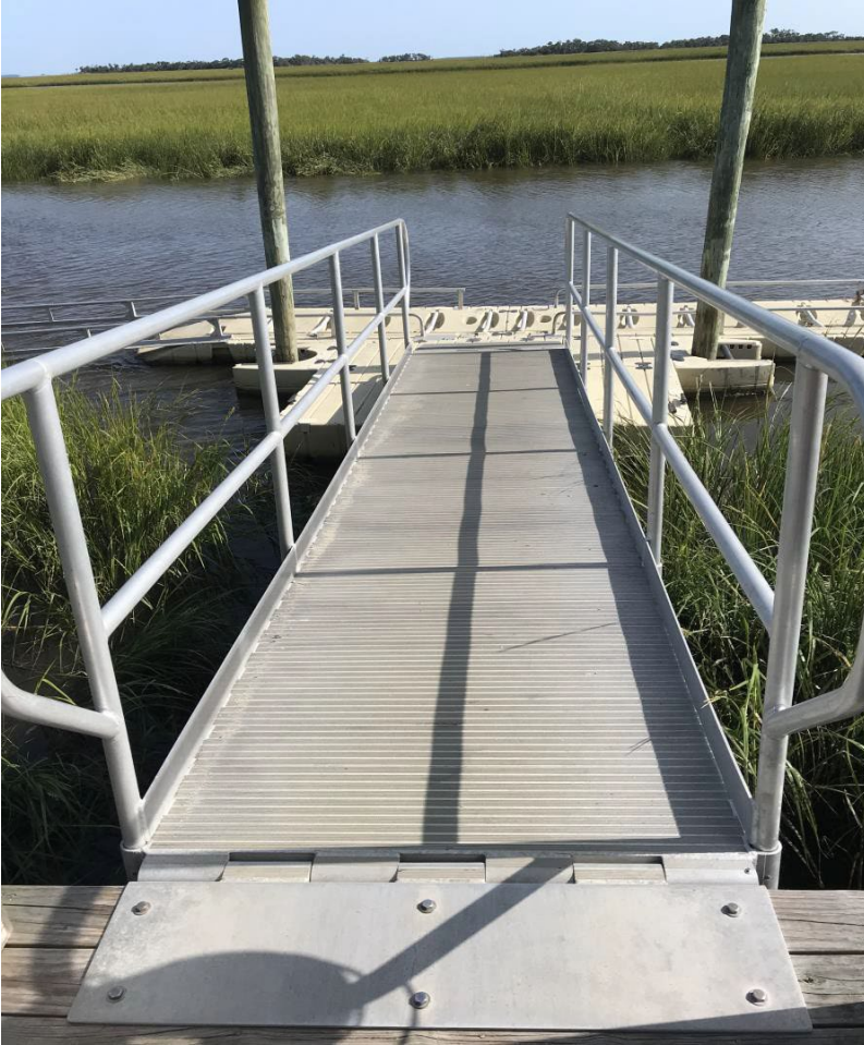
Dock and ramp to creek. Path to dock needs to be non-slip surface
