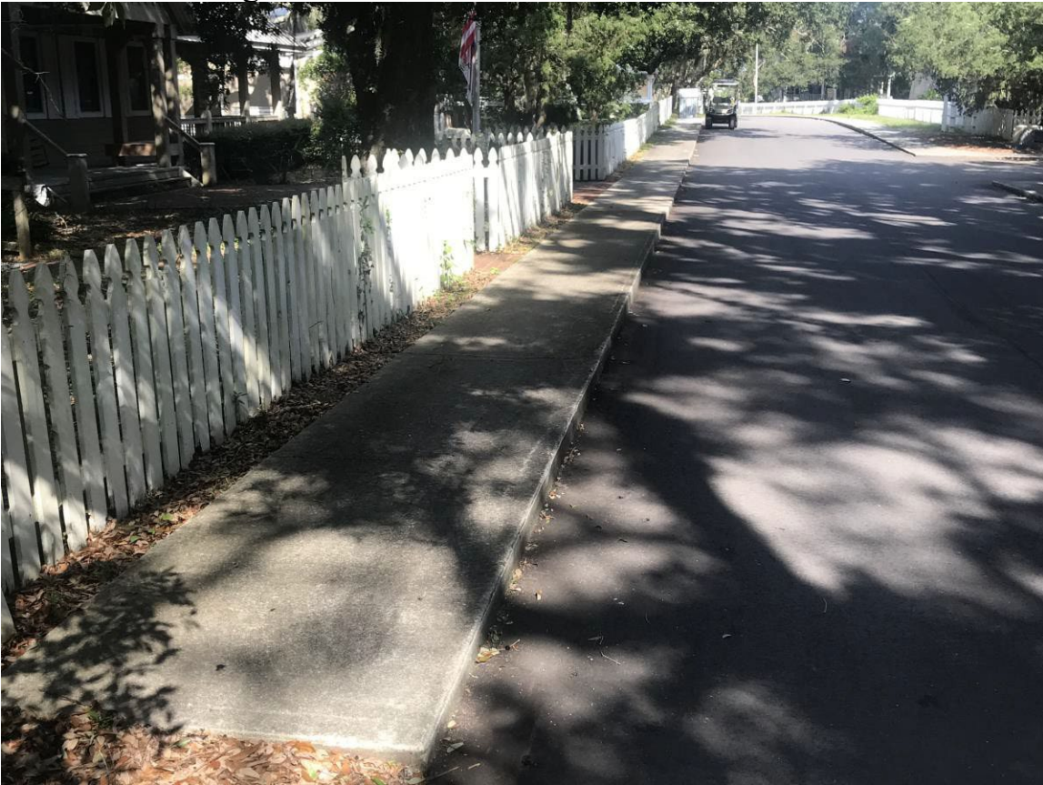
Area Where Curb cut was needed
